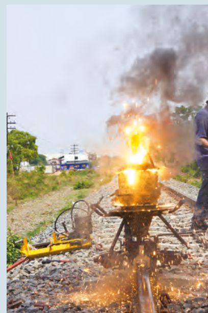
FIGURE 9.3.2 Thermite welding of railway tracks
